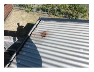
External cladding shows signs of rust and requires repair / repainting.
