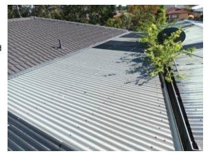
Damaged polyurethane sheeting requires repair.
